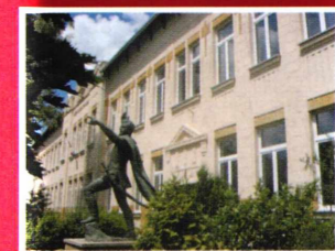
The renovated building of Grammar School.
